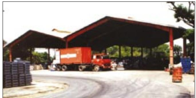
typical of Manila and Southeast Asia. Batteries are now stored under the cover of a purpose built 100 by 50 metre canopy. The new facility minimizes the risk of contamination to the surface water drainage system from battery acid. A surface drain that completely surrounds the storage area collects any leakage from the stored used batteries and the effluent is directed to the water treatment plant.
